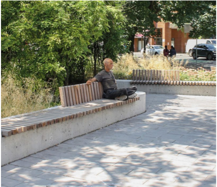
Seating retaining walls
