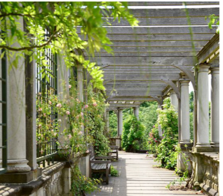
Reinstated heritage arbor structure with climbing plants
