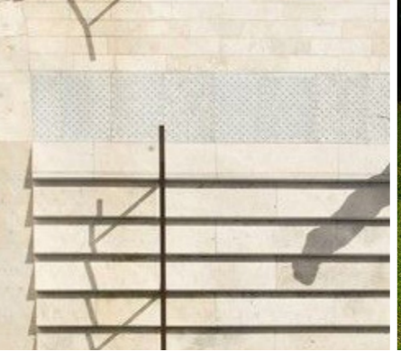
Compliant stair access
